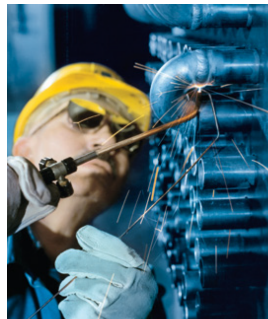
Gas welding work on heat exchanger.
