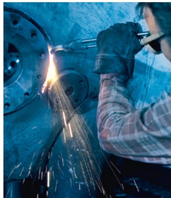
Gouging of the root for reverse side welding.
